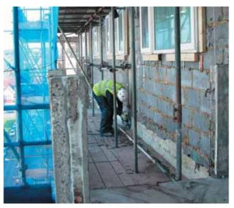
$\label{thm:carbonation} \mbox{ Loating was applied to Vertical Surfaces, and Zolpacryl Anti-carbonation Coating was applied to the Balcony Soffits \,. \,$
