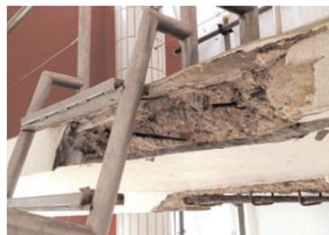
Once the defective concrete had been broken out, it became clear the main cause for the decay of the structure was due to the fixing bolts of the diving board and safety handrail. To prevent the same problem happening
