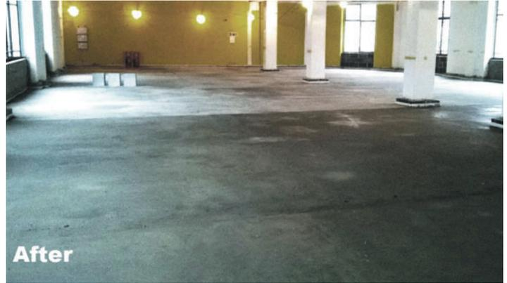
This was followed by the installation of 25mm of X21 hexatherm insulation and topped off with a floating/unbonded 30-40mm of Weber Floor 4310 incorporating Webers 4945 glass fibre net used within the screed as reinforcement.
