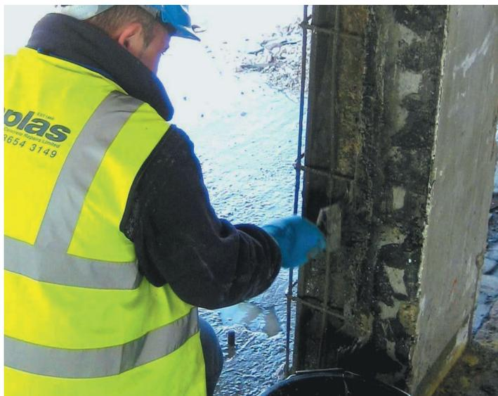
On completion of all repairs the columns were given a rendered finish using a Ronafix Polymer modified mortar. Using clean fresh water the columns were damped down until saturated removing any excess surface water followed by a Ronafix/Cement priming coat to the damp columns, and whilst the primer coat remained tacky a 10mm Ronafix Render was applied to all four sides of the columns. Prior to setting the Ronafix render was given a sponge finish.
