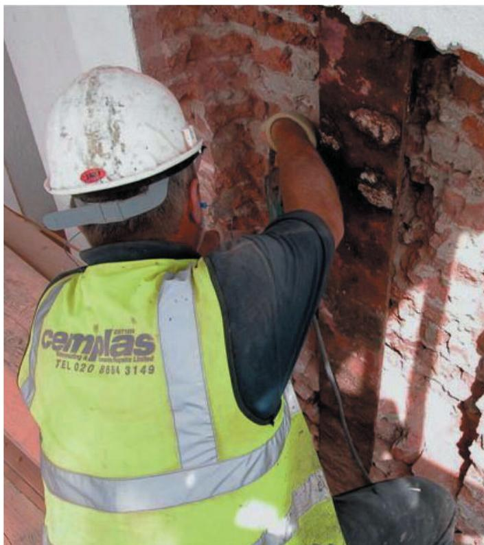
Cracks in masonry are the result of movement beyond that which can be accommodated by the construction materials. Buildings tend to crack where masonry is over-stressed and least restrained, such as at window and door openings or at corners. The movement is usually caused by variations in moisture content in the walls, or in the ground that supports them, temperature variations or by chemical reactions. Some movements are cyclic and reversible,
