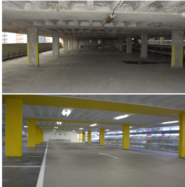
After: Deck Waterproofing
