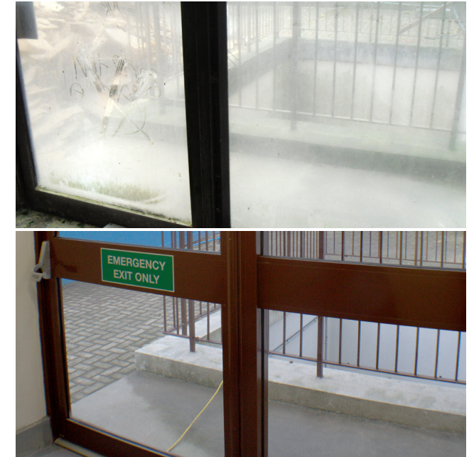
After: Pedestrian Entrances Replaced and Re-Glazed
