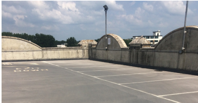
Before: Deck Waterproofing and Linemarking
