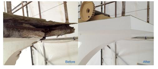
removed and re-fixed using a resin grout which would prevent water penetrating down through the bolts and into the structure. The handrail bolts which fell within the concrete repair areas were also removed and replaced with resin anchor fixings. The remaining handrail bolts were checked to ensure they weren't allowing water to pass through into the structure.
