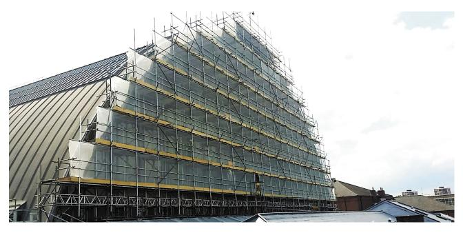
segments, chemical stripping the steel beams and repainting. Many of the projects undertaken at Olympia have had demanding access issues and in this instance Cemplas developed its own access arrangements by providing a scaffold which was built up from within the Exhibition Hall and cantilevered out.
