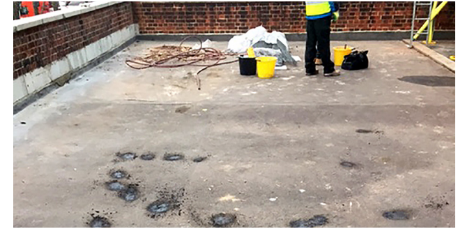
Before: Repair Substrate by Mechanical Abrasion
