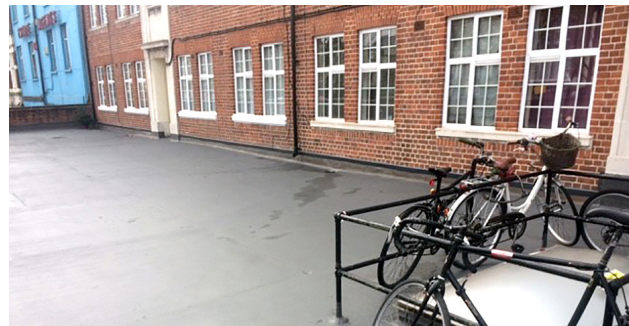
After: Slip-Resistant and Waterproof Surface
