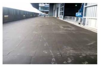
a two component, rubber/bitumen liquid applied waterproofing system with protection boards to provide a durable waterproofing and protection system capable of accepting various wearing surfaces subjected to both pedestrian and vehicular traffic.
