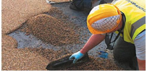
The works undertaken by Cemplas including laying an asphalt base course, followed by specialist Ronacrete's Ronadeck Resin Bound Aggregate Surfacing System, including the fitting of aluminium angle trims.
