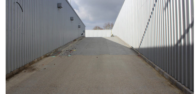
Before: Re-waterproofing Access Ramps
