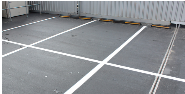
After: Mechanical Movement Joint
