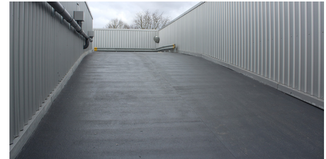
After: Re-waterproofing Access Ramps
