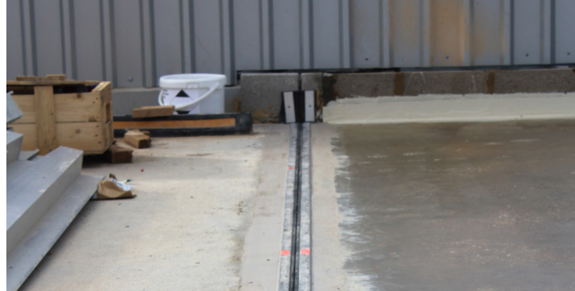
Before: Mechanical Movement Joint
