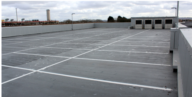
After: Re-waterproofing Top Deck
