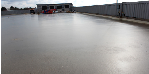
Before: Re-waterproofing Top Deck
