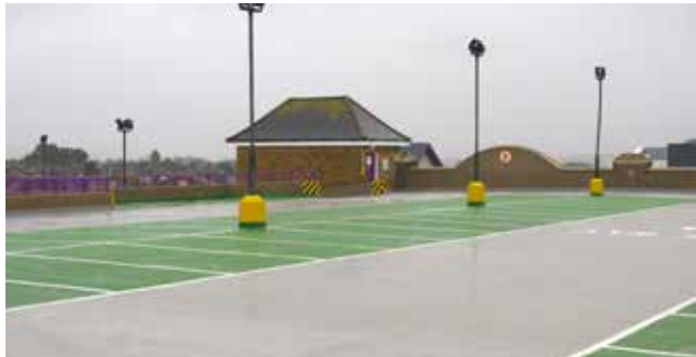
After: Deck Waterproofing and Linemarking
