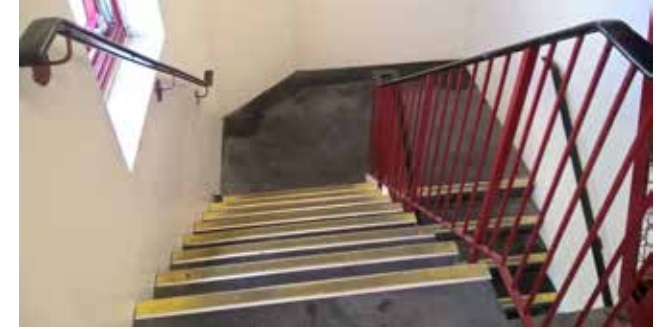
Before: Stairwell Refurbishment
