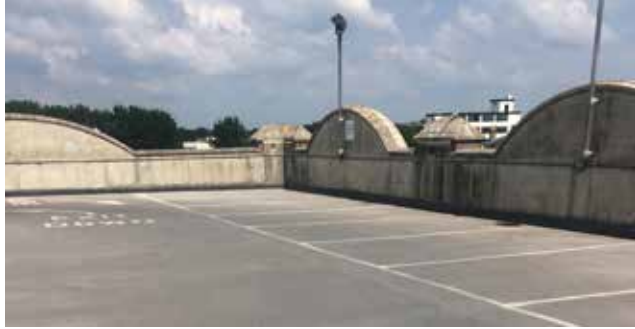
Before: Deck Waterproofing and Linemarking
