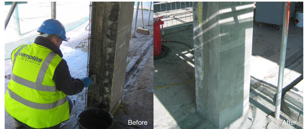
**Faced with the task of the £25 million renovation of the Museum of Bristol made possible due to a £11.3 million Heritage Lottery Fund grant, HBG Construction Ltd appointed specialist contractors Cemplas Waterproofing and Concrete Repairs Limited to undertake in excess of £100,000 of remedial concrete repairs and protective coatings to all of the all concrete surfaces, including beams, columns, soffits and fascias.**
