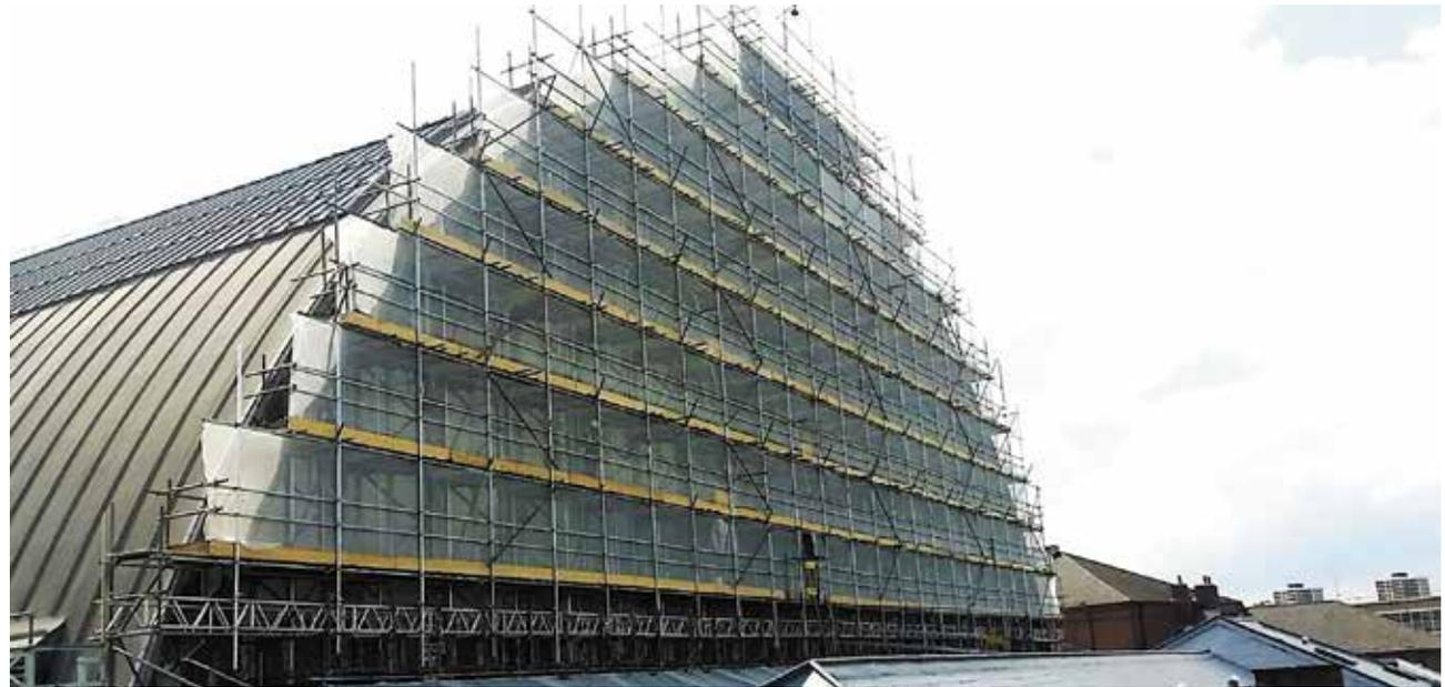
segments, chemical stripping the steel beams and repainting. Many of the projects undertaken at Olympia have had demanding access issues and in this instance Cemplas developed its own access arrangements by providing a scaffold which was built up from within the Exhibition Hall and cantilevered out.
