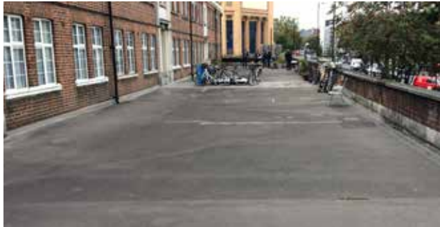
Before: Balcony Walkway Resurfacing
