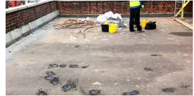
Before: Repair Substrate by Mechanical Abrasion
