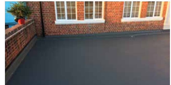
After: Repair Substrate by Mechanical Abrasion
