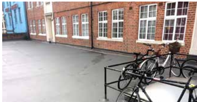
After: Slip-Resistant and Waterproof Surface
