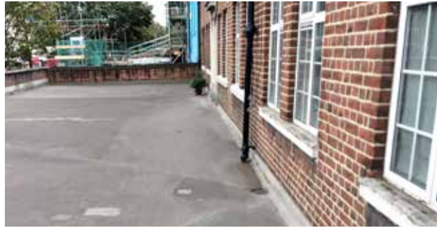
Before: Slip-Resistant and Waterproof Surface
