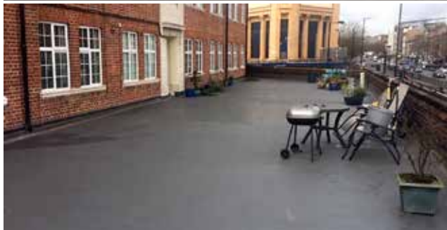
After: Balcony Walkway Resurfacing
