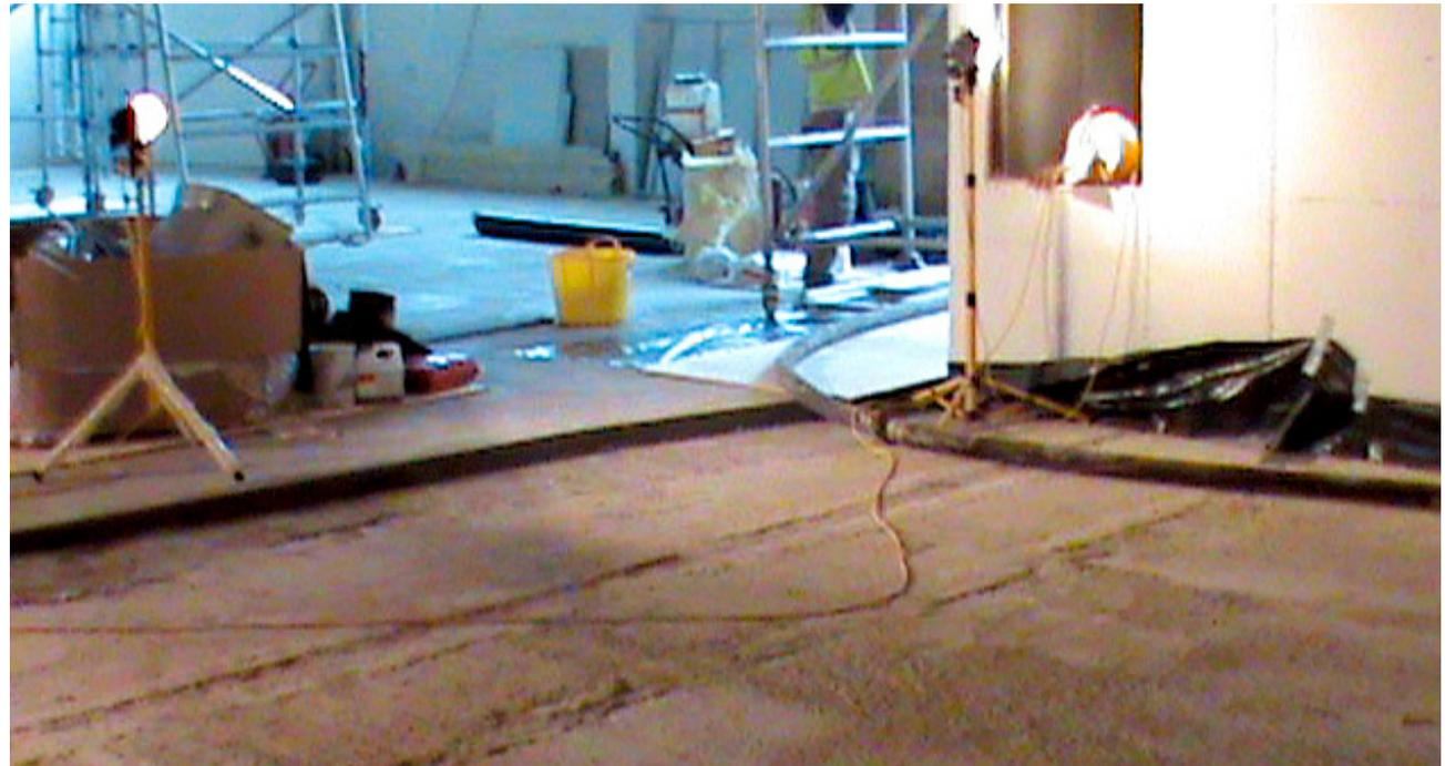
On completion of the new floor surface, and after a full curing period the main floor was handed over to the main contractor who began the fitting out process.
