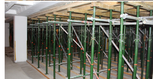
Propping during Re-casting
