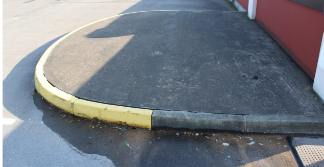
Before: Damaged kerbs
