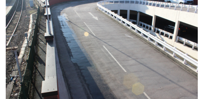
Before: Damaged asphalt on ramps
