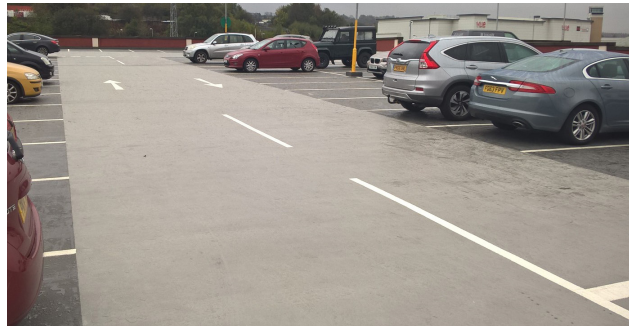
After: Decks re-waterproofed
