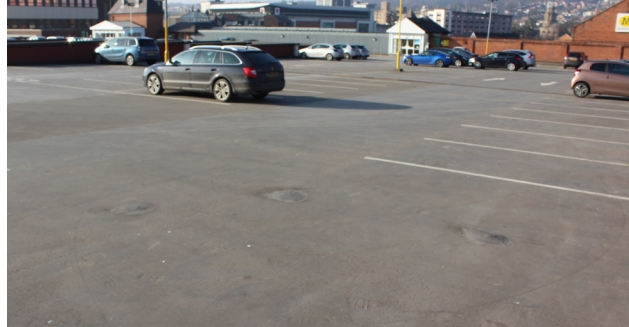
Before: Blistered and split asphalt
