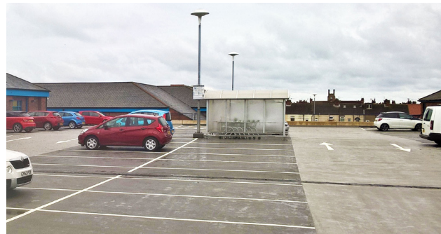
After: Movement joints installed
