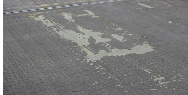
Before: Delaminated surface
