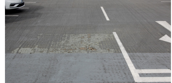
Before: Worn out waterproofing
