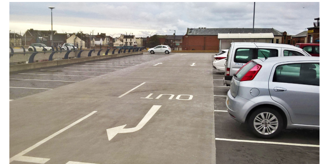
After: Decks re-waterproofed
