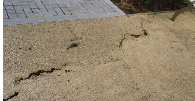
Before: Sub-Base Repairs Required
