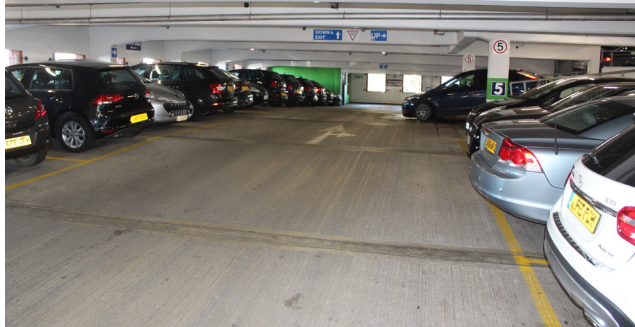
Before: Unprotected Concrete Decking
