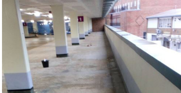
Before: Failed decking
