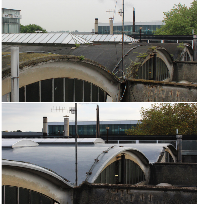
After: Roof Re-waterproofed
