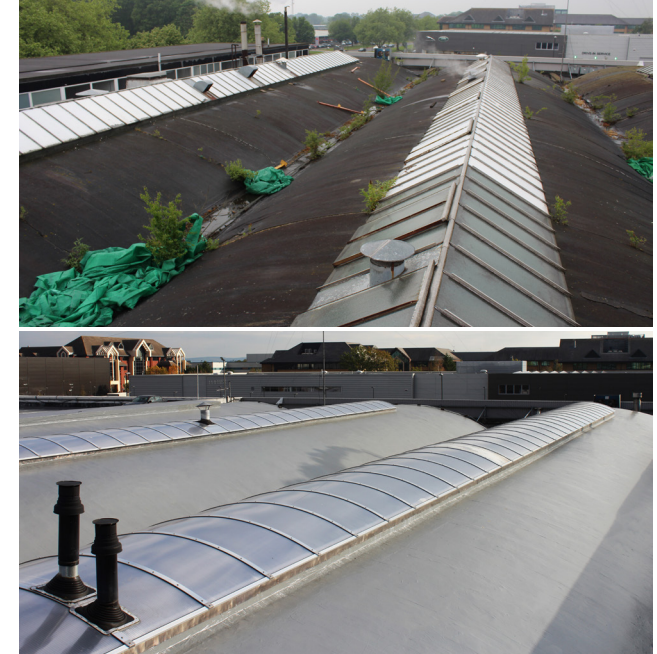
After: Watertight Overlay of Roof
