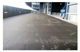
a two component, rubber/bitumen liquid applied waterproofing system with protection boards to provide a durable waterproofing and protection system capable of accepting various wearing surfaces subjected to both pedestrian and vehicular traffic.
