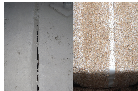
Hypalon strip over movement joints
