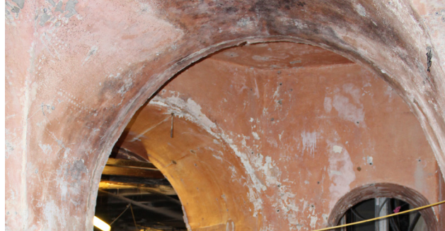
Before: Long term Water Ingress Damage
