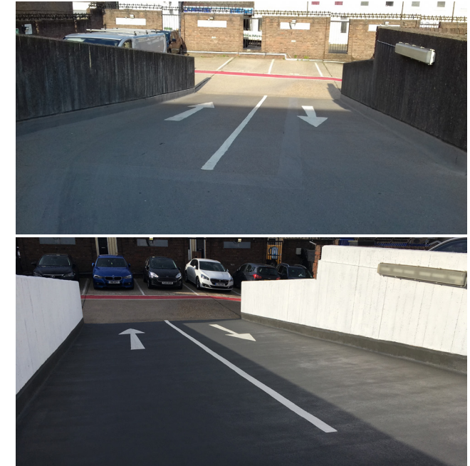
After: Fully Protected Ramps
