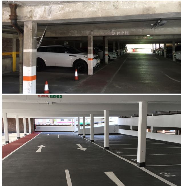
After: Light & Bright Interior Improvements
