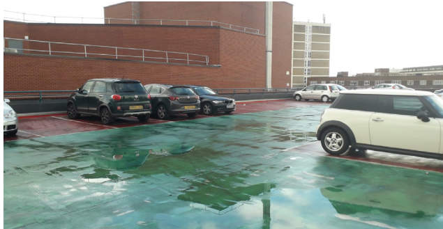
Before: Existing Waterproofing Beyond Service Life
