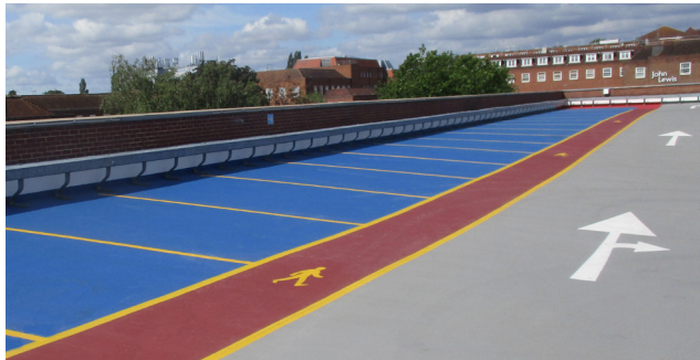
After: Re-waterproofed in Contrasting Colours
