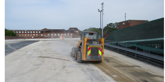
During: Removal of Existing Waterproofing
