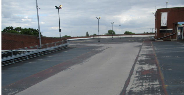
Before: Existing Waterproofing > 15 Years Old
