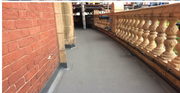
After: Fully Re-waterproofed Walkways
