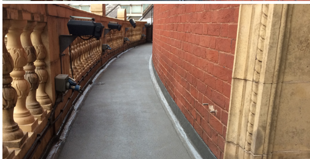
After: Seamless (Joint-free) Application
