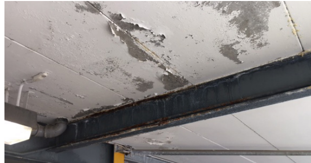
Before: Damaged Soffits from Water Ingress
