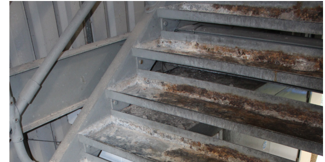
Before: Badly Corroding Stair Treads
