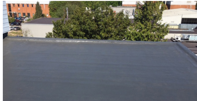
After: Watertight Overlay of Roof
