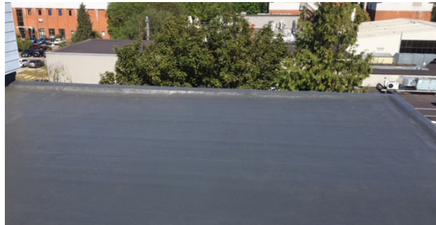
After: Watertight Overlay of Roof
