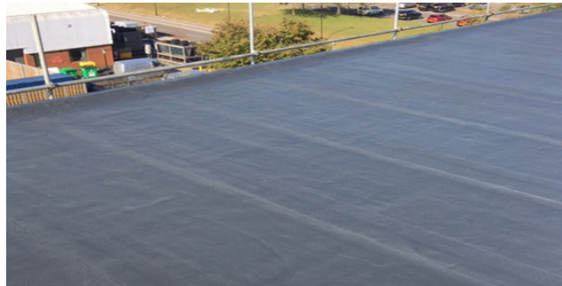
After: Cold, Liquid-Applied Application
