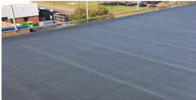
After: Cold, Liquid-Applied Application
