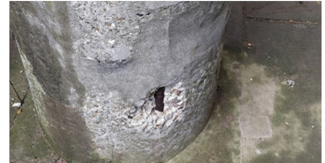
Before: Concrete Delamination
