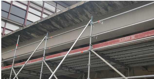
After: Fully Protected Beams
