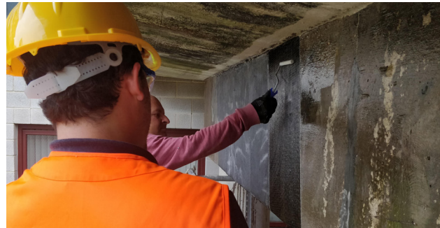
During: Application of Mapeband
