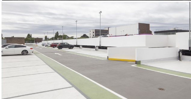
After: Fully Rejuvenated Decks & Parapets
