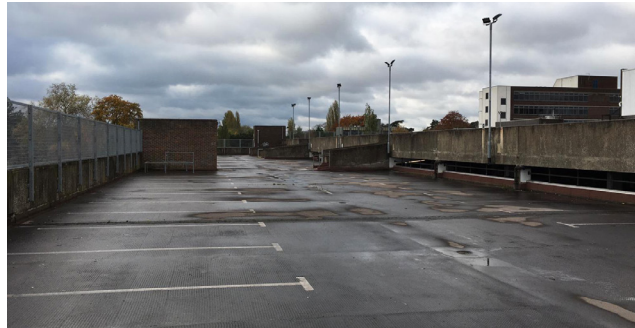
Before: Existing Top Decks & Parapets
