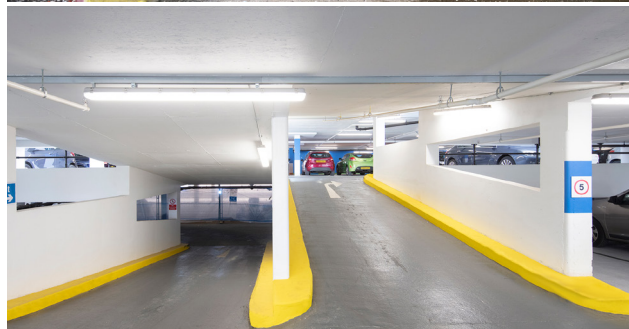
After: Refurbished Ramps
