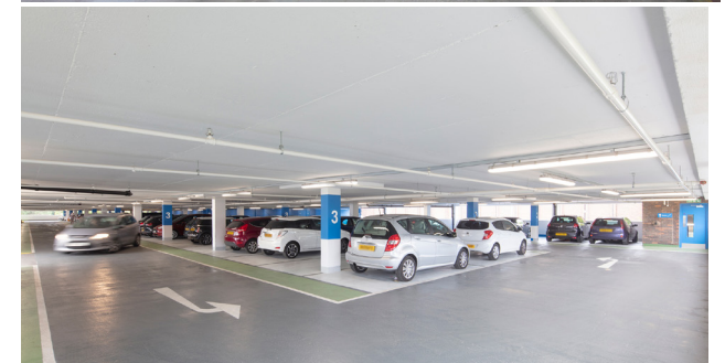
After: Light & Bright Interior Improvements
