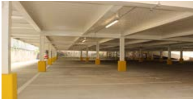
After: Structure Repaired
