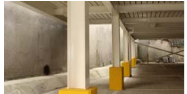
After: New Intumescent Coatings Applied
