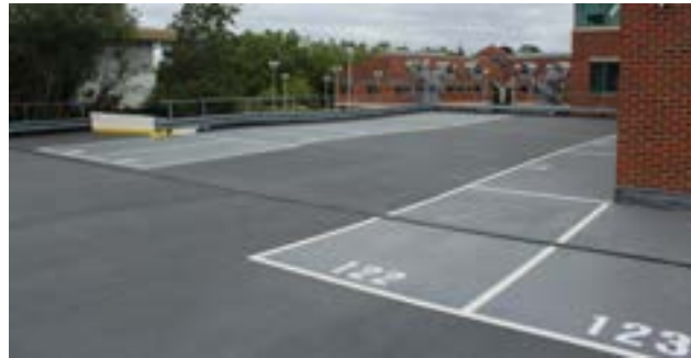
After: Fully Watertight Parking Deck
