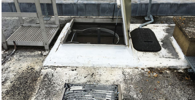
Before: Leaking Entrance Hatch
