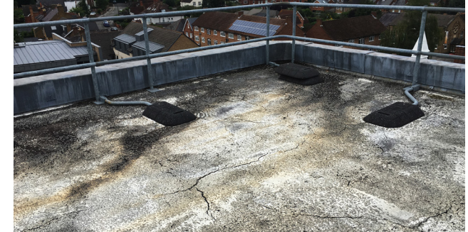
Before: Split & Damaged Asphalt
