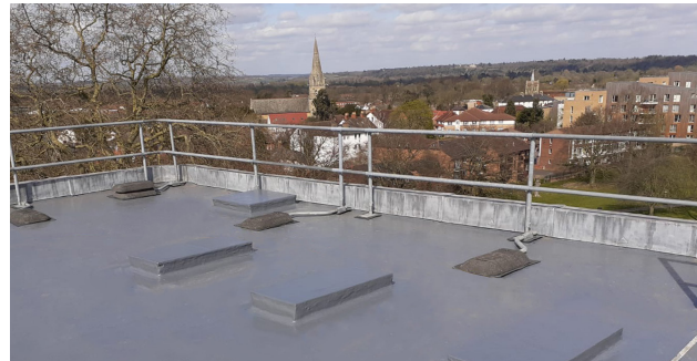
After: Rooflight Capped Off
