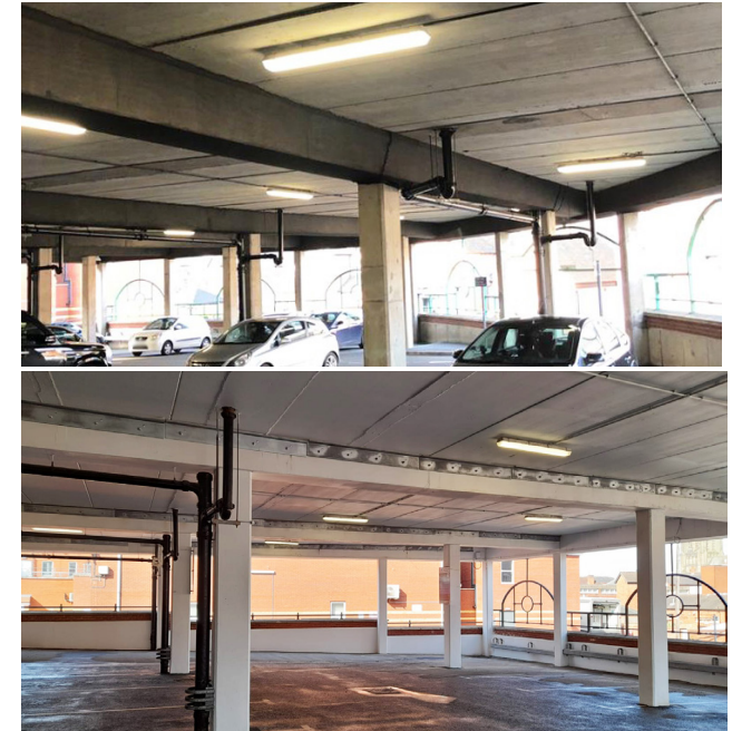
After: Repaired & Protected Structural Beams & Columns
