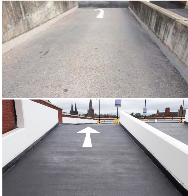
After: Protected Ramps
