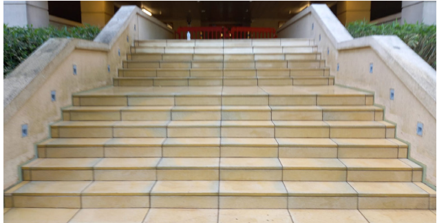
After: Steps Fully Waterproofed
