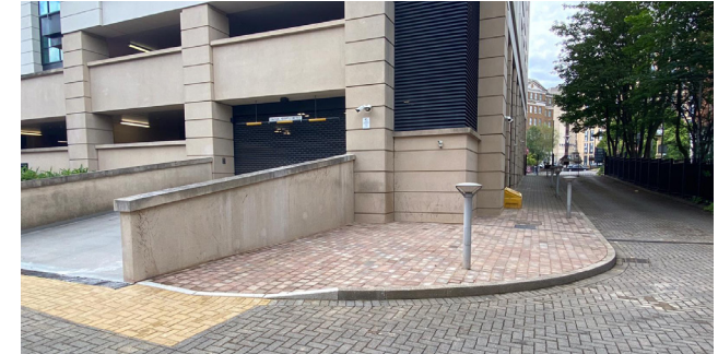
After: Exit Ramp Watertight
