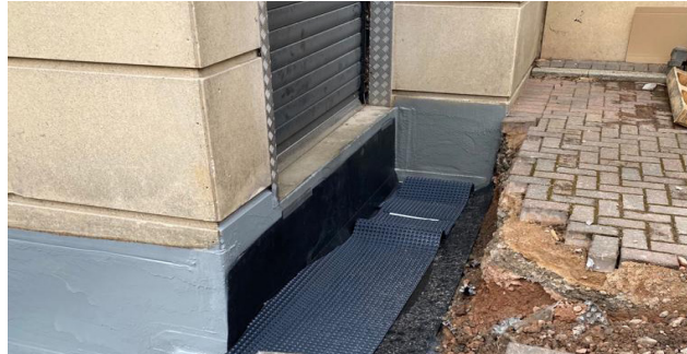
During: Drainage Installed
