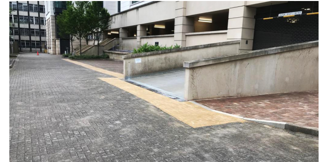
After: New Pedestrian Walkway
