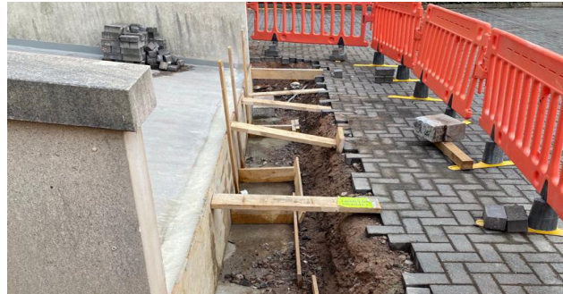
During: Block Paving Removal & Excavation
