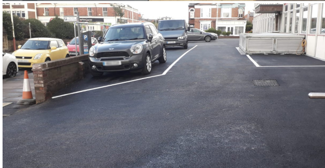
After: Fully Protected Car Park & External Landscaped Areas
