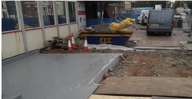
During: Waterproofing Detail To Basement Structure
