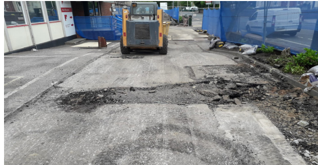
During: Removal of Existing Coatings
