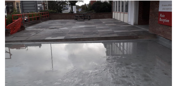
During: Seating Area Waterproofed
