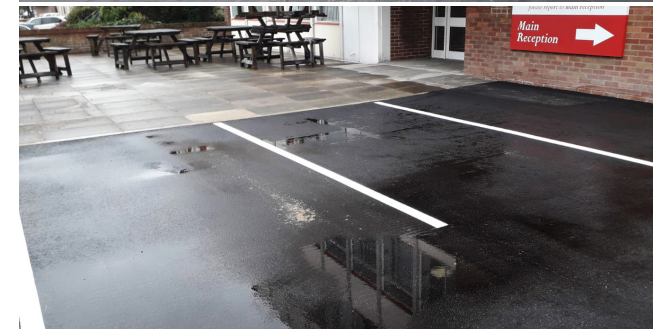
After: Car Park Reinstated
