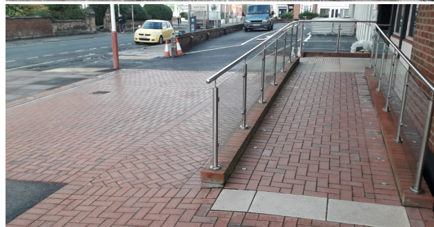
After: Improved Entrance To The Car Park
