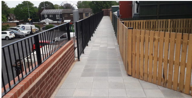
After: Fully Refurbished Walkways
