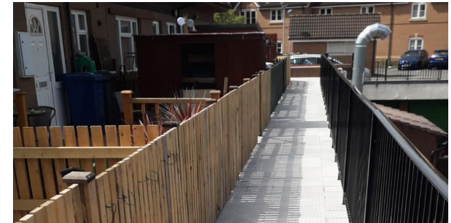
After: Walkways Enhanced & Upgraded
