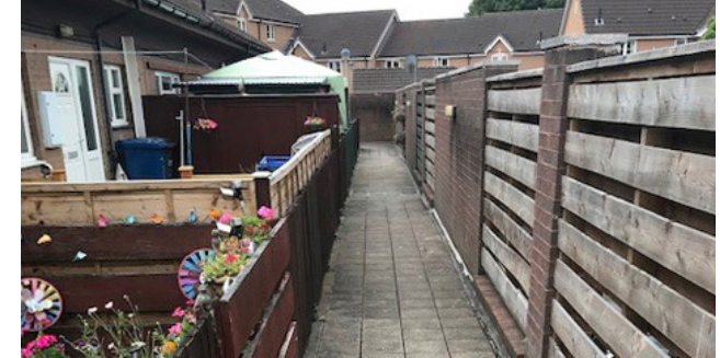
Before: General Poor Condition
