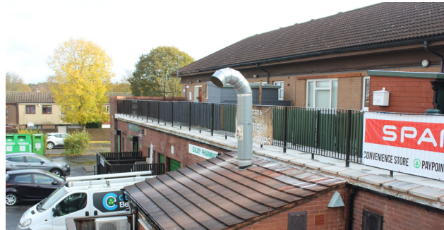
After: Replacement Balustrading Installed
