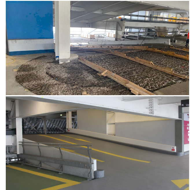
After: Precisely Reprofiled Ramps
