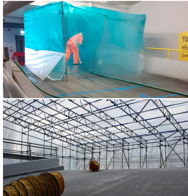
During: Scaffolding & Sheeting for 'Tenting In' on Exposed Top Deck
