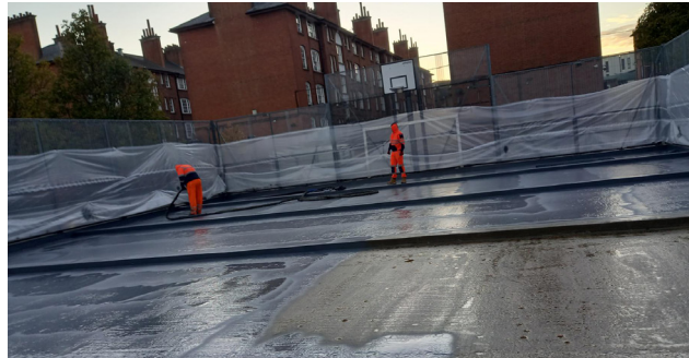
During: Application of Spray Applied Waterproofing
