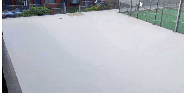
After: Fully Protected Courtyard & Walkways
