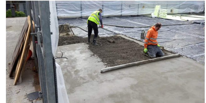
During: Screeding Reinstatement
