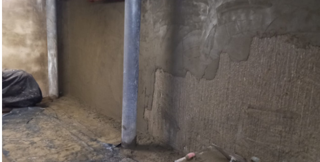
During: Cementitious Render To The Basement Car Park
