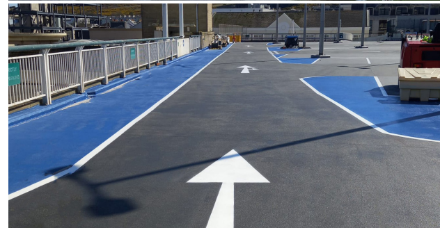
After: Fully Protected & Watertight Decks
