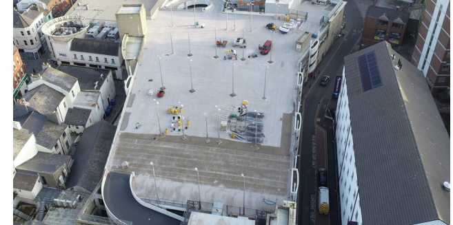
During: Application Of Fully Reinforced Waterproofing
