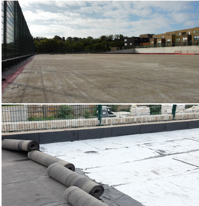
During: Sand Faced Capping Sheet Installation
