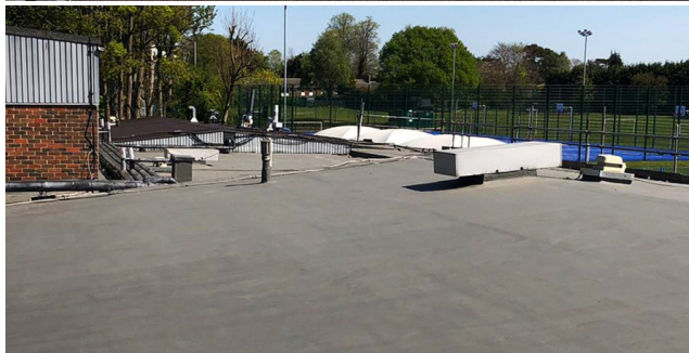
After: Cold, Liquid-Applied Application
