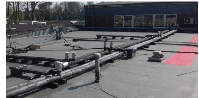
After: Watertight Overlay of School Roof
