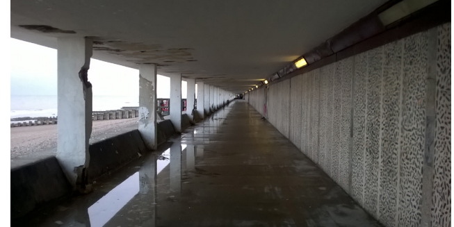
Before: Columns and Soffits Unprotected
