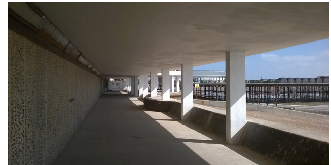
After: Protective Coatings Applied
