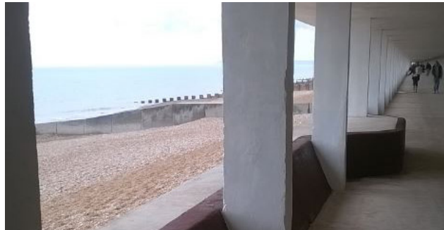
After: Extensive Repairs Carried Out
