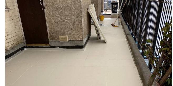
During: Tapered Insulation
