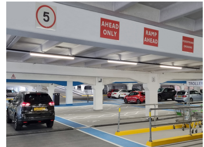
After: Light & Bright Interior Improvements
