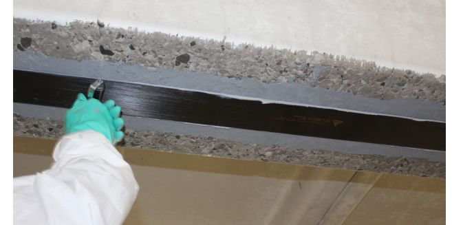
During: Application of Carbon Fibre
