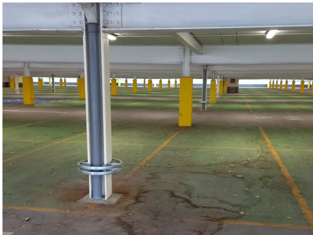
During: Repaired & Protected Structural Steel Columns
